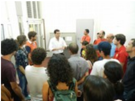
Figure 3.40 Visit to the Alqueva Hydro Power Plant, guided by André Silva.
